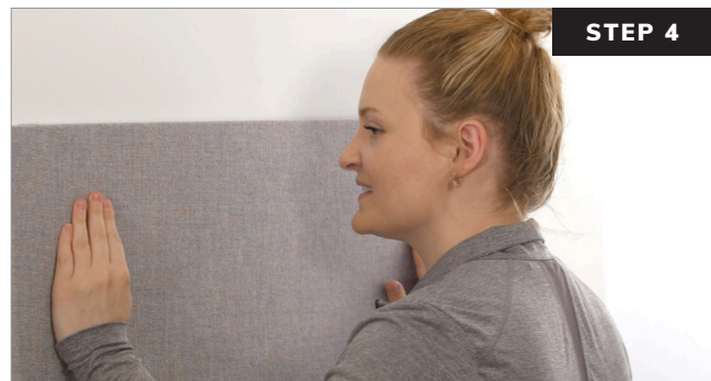
Push panel against wall to mark anchor locations.
