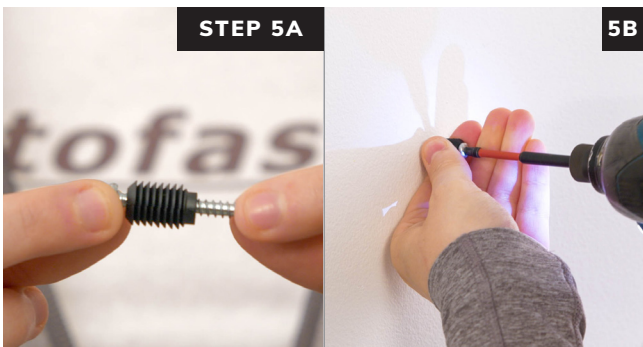
Screw ratchets to wall at marked locations. Flat end of ratchet goes against the wall, curved end faces out.
