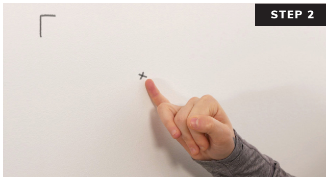
Mark the locations on the wall where the black ratchets will be installed in Step 3. For help with the number and placement of anchors, contact Rotofast.
